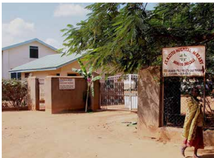
The entrance to St. Kizito Hospital in Matany
