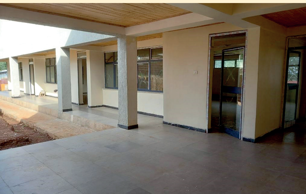
Ongoing building work
